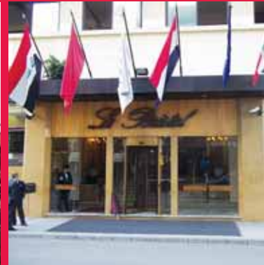
Structural Rehabilitation of "Le Bristol Hotel", Beirut, Lebanon
