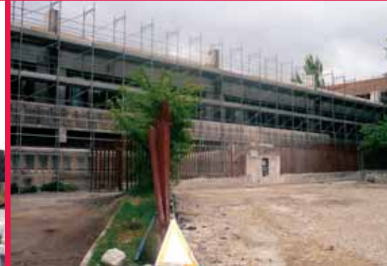
Structural repair and rehabilitation of High Court (Tribunale) building, Italy
