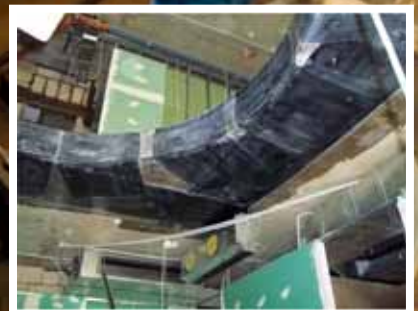
Upgrading a circular opening of Park Palace Pronivias, Lebanon
