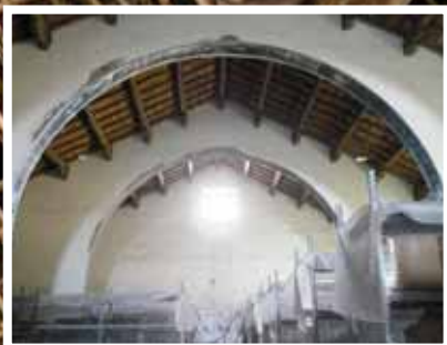
Strengthening and Repair of masonry arches, Tuscany, Italy
