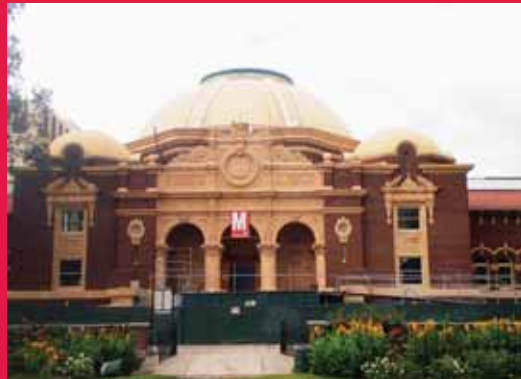
Rehabilitation and Strengthening of Natural History Museum, Los Angeles, California
