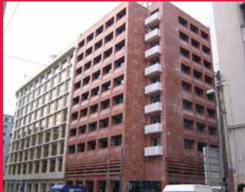
Seismic and Fire-Resistant Upgrade of Hotel "Kaningos 21", Athens, Greece
