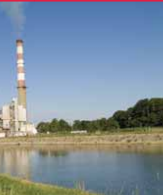
Installation of a large diameter steel Injection Pipe, Yorktown.
