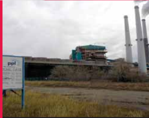
Rehabilitation & Strengthening of over 100 linear feet of six 72" diam. PCCP of PPL Montana
