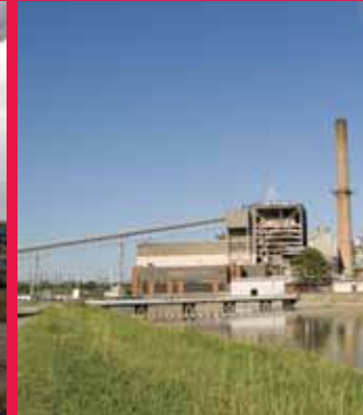
Strengthening and Rehabilitation of pipe of the power plant Dominion Energy
