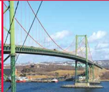
Rehabilitation of corroded members (PT cable) of MacKay Bridge , Canada
