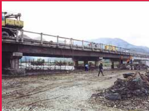
Structural Strengthening of Xerias River Motorway bridge , Argirokastro, Albania
