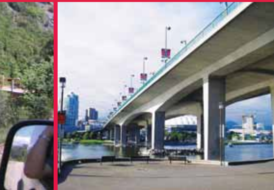
Seismic upgrade Knight Street Bridge , Vancouver, Canada
